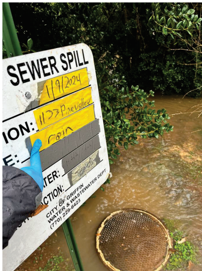
Figure No. 2: Manhole No. 1
